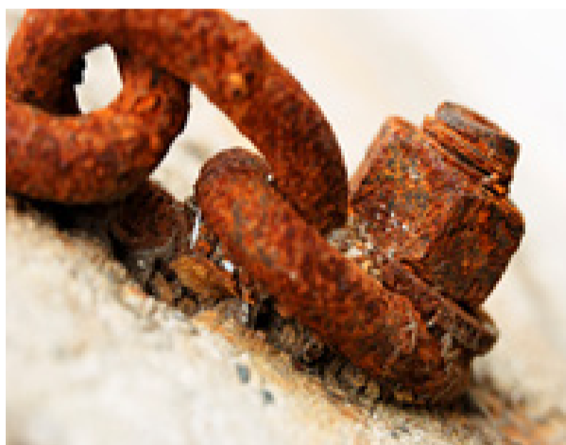
Figure 1: Cast iron metal turns rusty when oxidized. Different chemicals can cause this, such as hydrogen, oxygen, salt, or other acids and corrosives.
