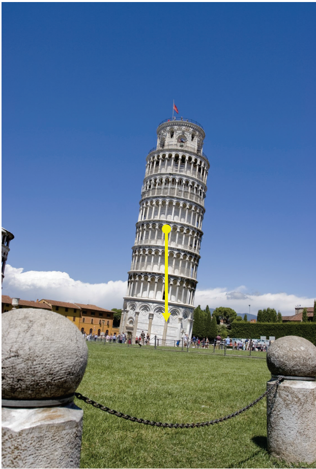
Figure 2: The Leaning Tower of Pisa.
